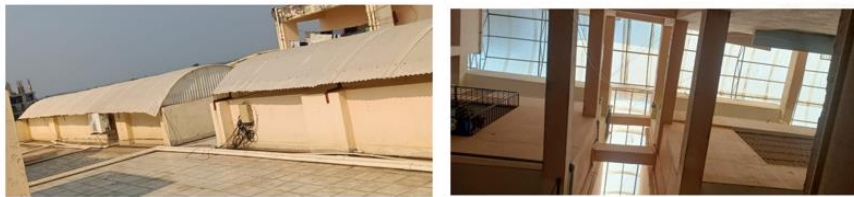
(a)Roof top vent with shading
