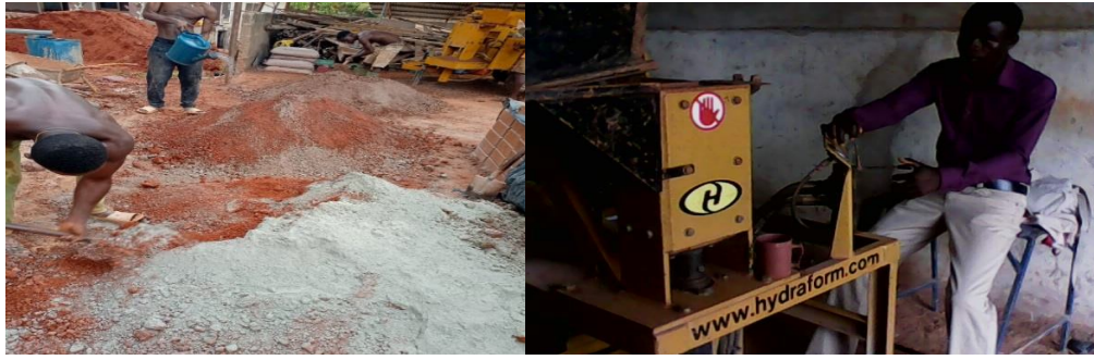
Figure 6: Mixing and moulding with hydraform machine set up
