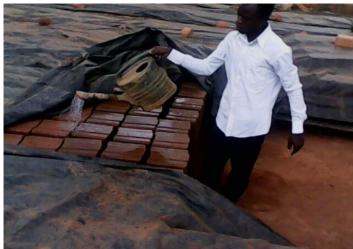
Figure 7: Curing and storage of compressed laterite interlocking blocks.
