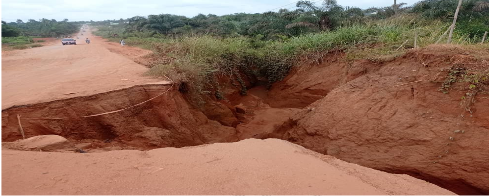
Figure 1.: Field Observation Showing Soil Loss impacted site in Study Area Source: Authors Field Work (2022)
